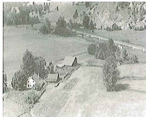
Brent's Grist Mill buildings at original location
